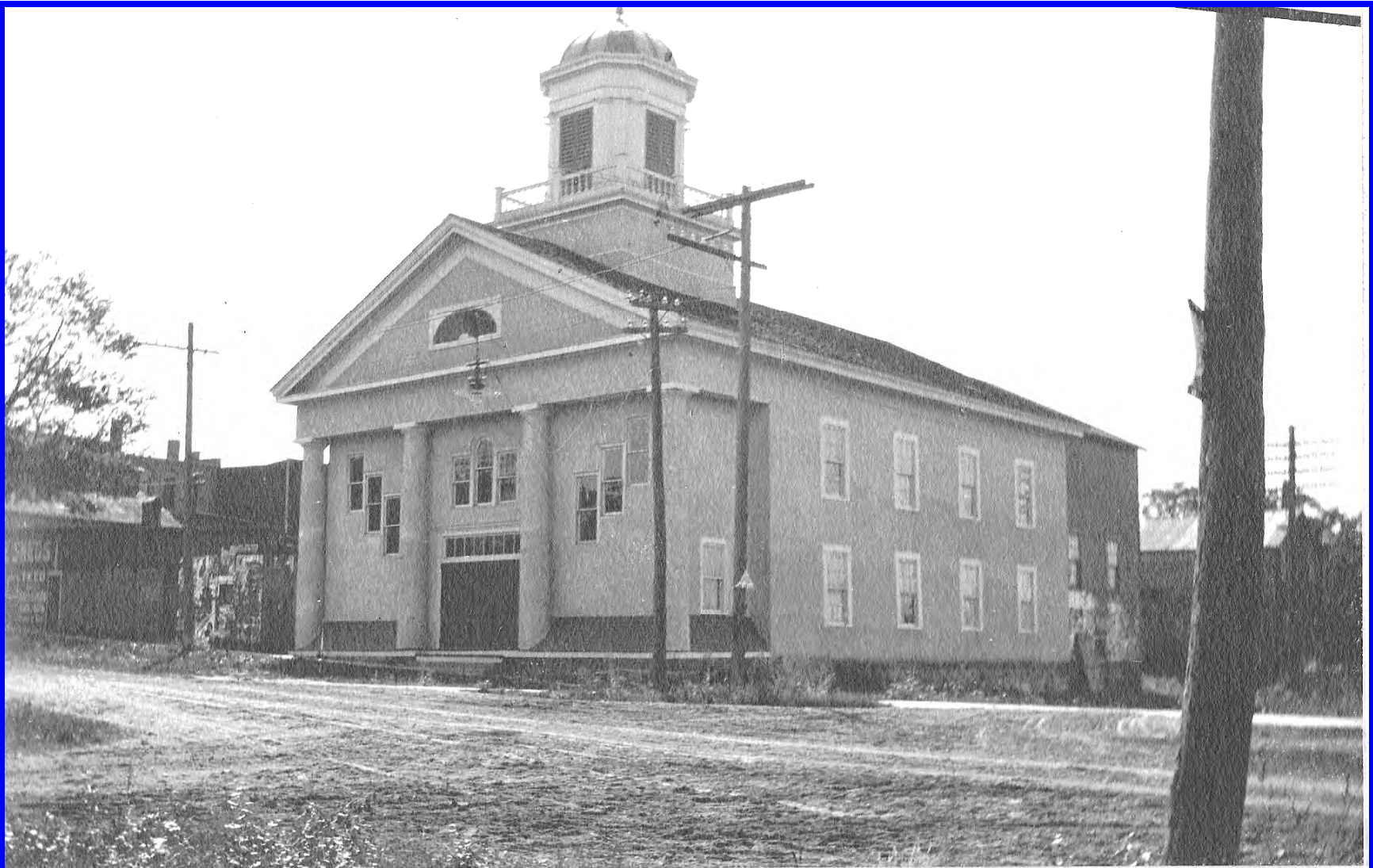
Old Court House on W. State St. Now used as Movie Picture House Built 18
